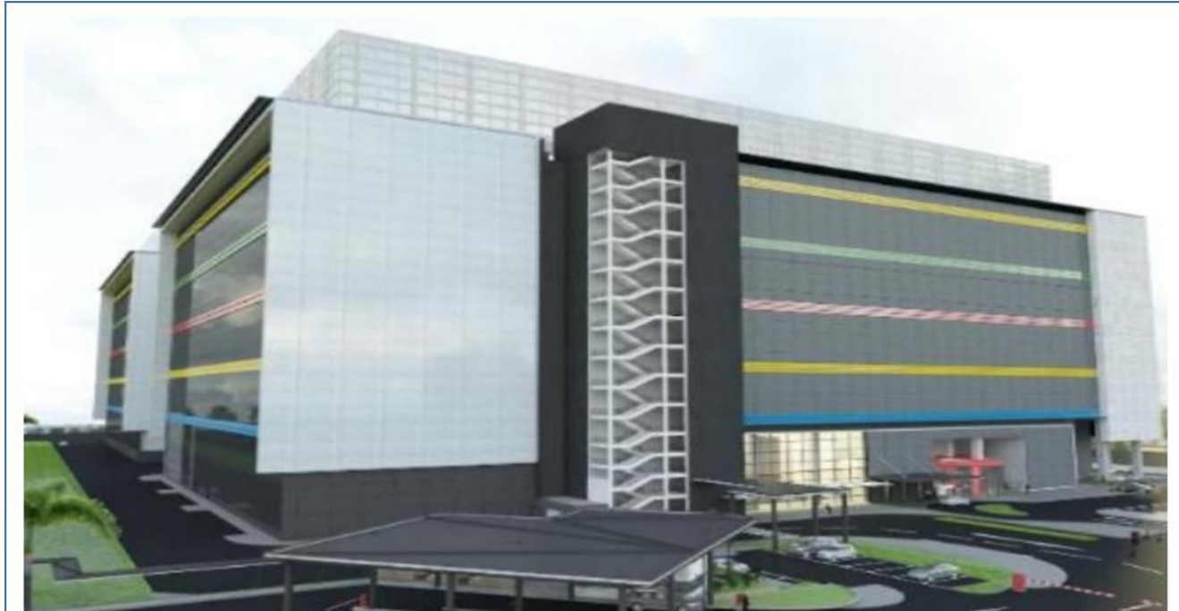
Google said the third data centre, which is expected to come online in 2020, will be built on a plot of land the size of the first and second centres combined. PHOTO: GOOGLE
